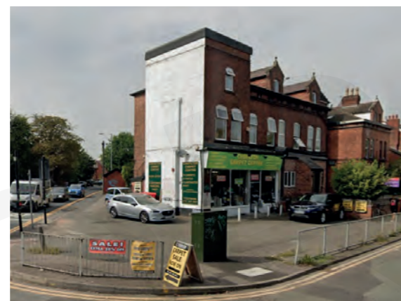
Example blank façades
