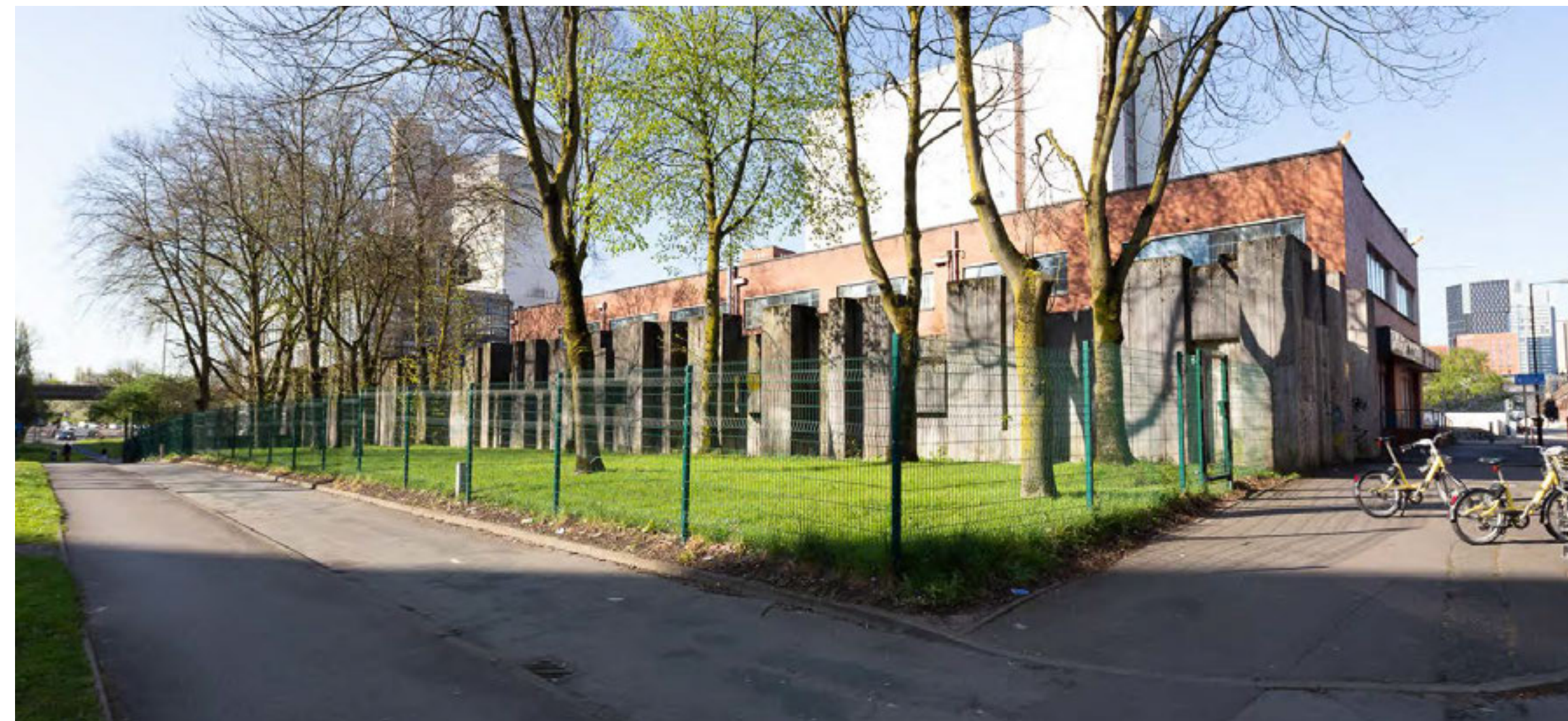
Image: Photo of Hollaway Wall looking west from London Road
