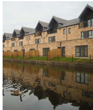
The Dob Brook Close scheme in Newton Heath, completed by Guinness Partnership in October 2022
