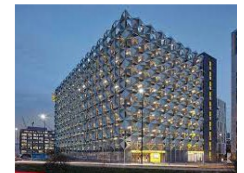
Stanley Street Car Park, Salford
